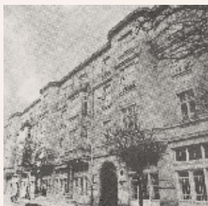
General view of the building from the 1970s. LSA.
