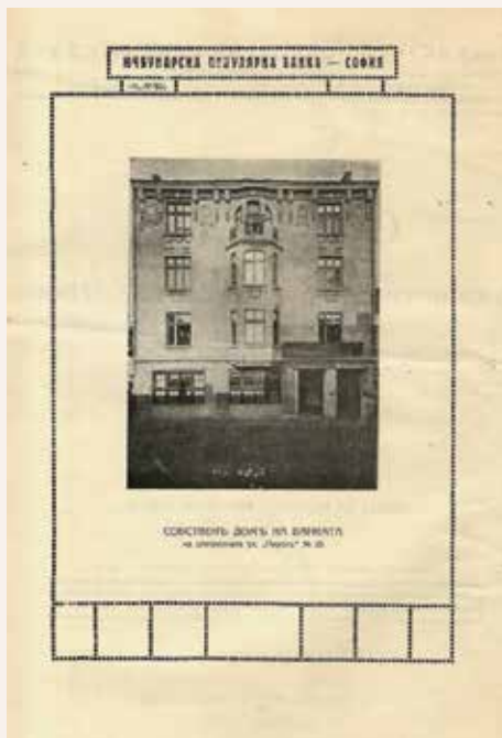
The Yuchbunarska Popular Bank building. The photograph was published in 1937 in the bank's report. Source: https://alba-books.com
